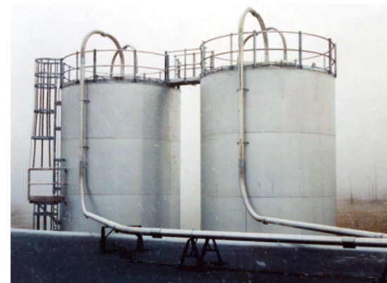
Tank & vessel construction
